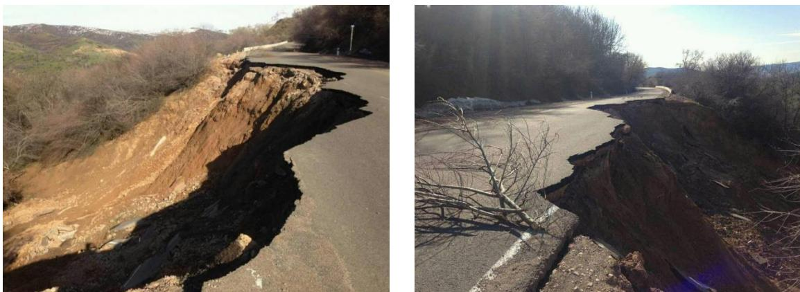
Figure 1. Landslides on the area of the road
